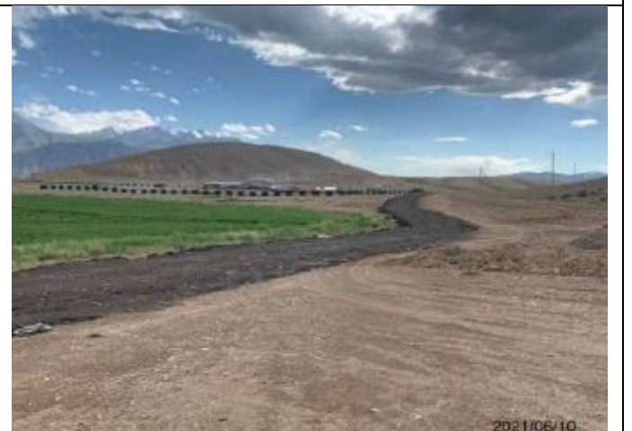
Photo 55. Lot 2. Old asphalt, to prevent dust formation, laid on the technological ground road to Crushing plant.
