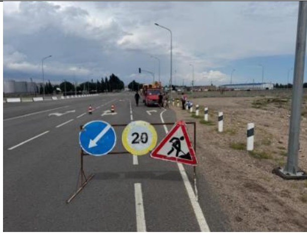
Photo 11. Dismantling of signal posts for the installation of a guardrail. August 2025.
