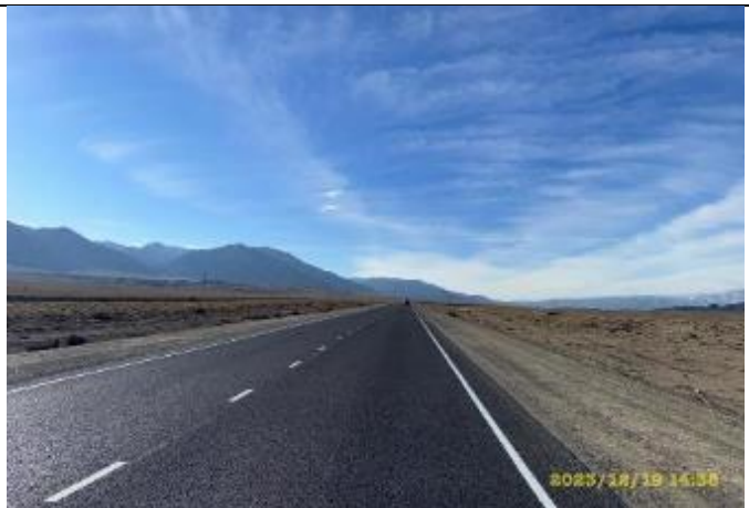
Photo 78. Lot 1: Road with new asphalt pavement.
