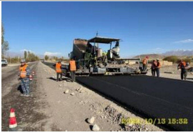
Photo 74. Lot 2. Binder course paving km 87+100.
