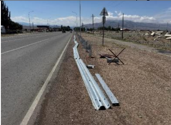
Photos 7, 8. Lot 1. Installation of barrier fences July 2025.
