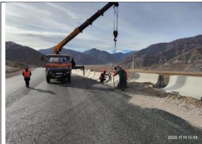
Photo 109. Installation of parapets on 40+700-40+870 RHS.
