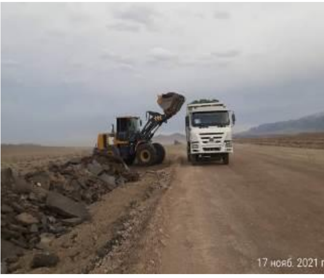
Photo 42. Scarifying and removal of old asphalt at km. 28+200-28+700.
