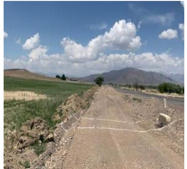
Lot 2. Photo 8. Area after clearing of stump and uprooted stumps.
