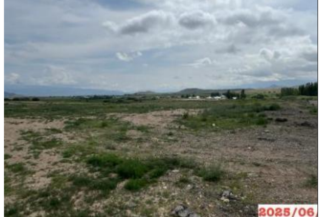
Photo 29. Lot 2. Old asphalt dump at km 89+093 after its reclamation
