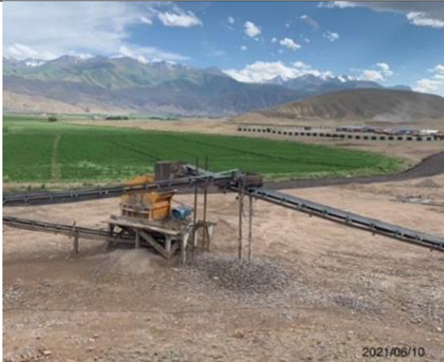
Photo 131. Location of the stone crushing plant production base and Contractor's camp.
