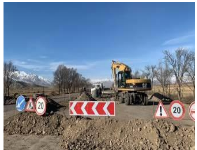
Photo 98. Lot 1. Compaction of soil backfill of culvert at km 20+670.
