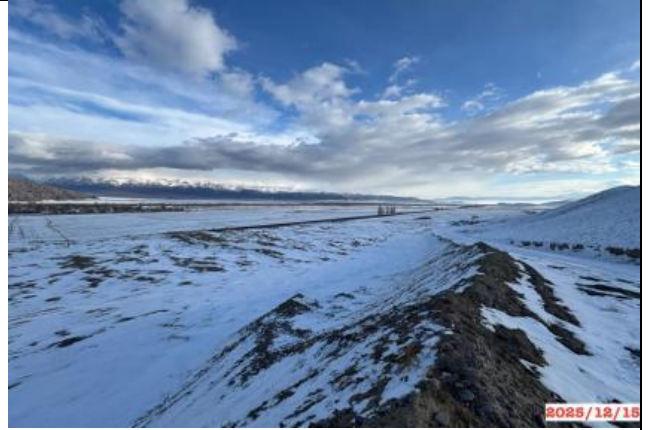
Photo 27. Lot 2. Reclaimed spoil dump of unsuitable soil at km 80+900 in winter. December 2025.
