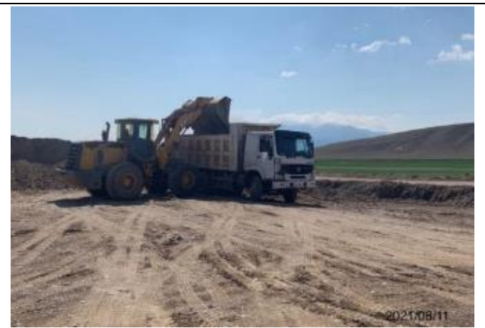
Photo 34. Quarry at km. 81+200, loading of moistened material.
