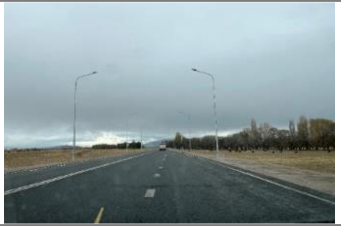
Photo 81. Lot 2. Road with new asphalt pavement.
