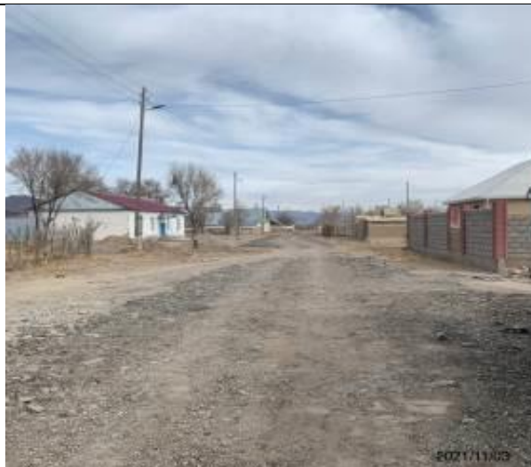
Photo 60. Improvement of internal roads in Epkin village.
