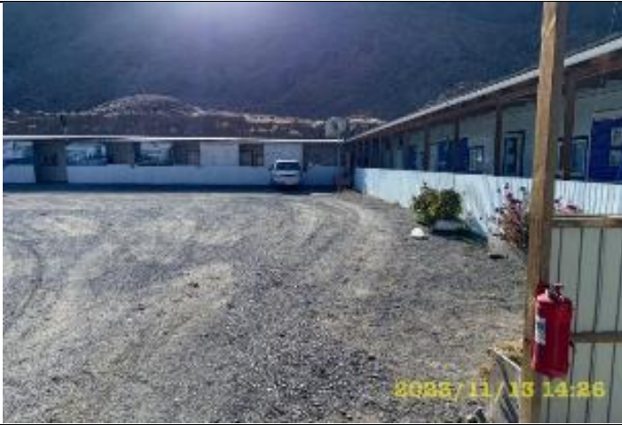
Photo 121 Lot 1. Subcontractor's accommodation camp.
