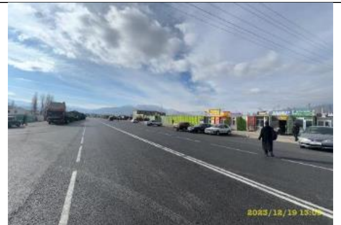
Photo 79. Lot 1. Road with new asphalt pavement.
