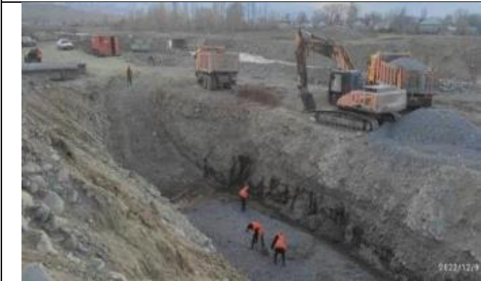
Photo 88. Bridge construction at km 65+410. Installation of the foundation for the bridge piers.
