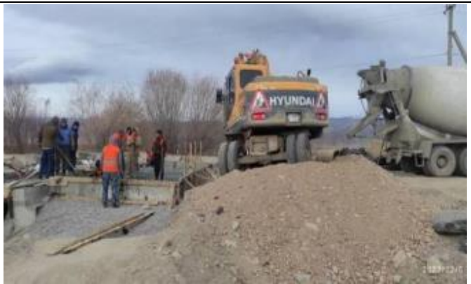
Photo 89. Concrete pouring of transition slab 1 km 68+044.
