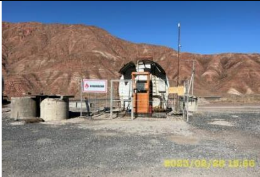
Photo 118. Lot 1. Sanitary condition of filling station territory.
