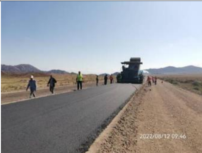
Photo 76. Lot 1. Binder course paving on km 17+230 - km 17+500.
