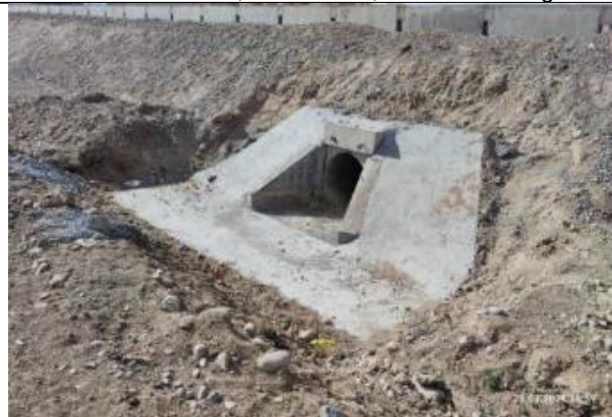
Photo 105. Lot 2. Construction of reinforcement at culvert inlet, km.88+692
