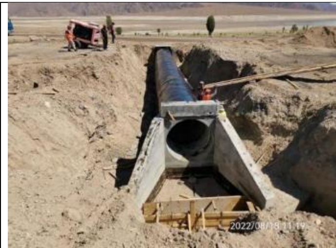
Photo 97. Lot 1. Completed installation and waterproofing of culvert at 37+161.
