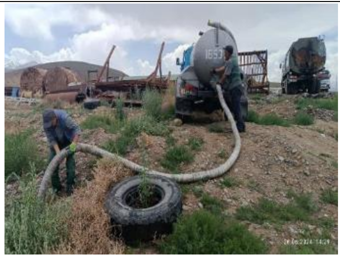
Photo 71. Lot 1. Removal of liquid wastewater from Contractor's camp.
