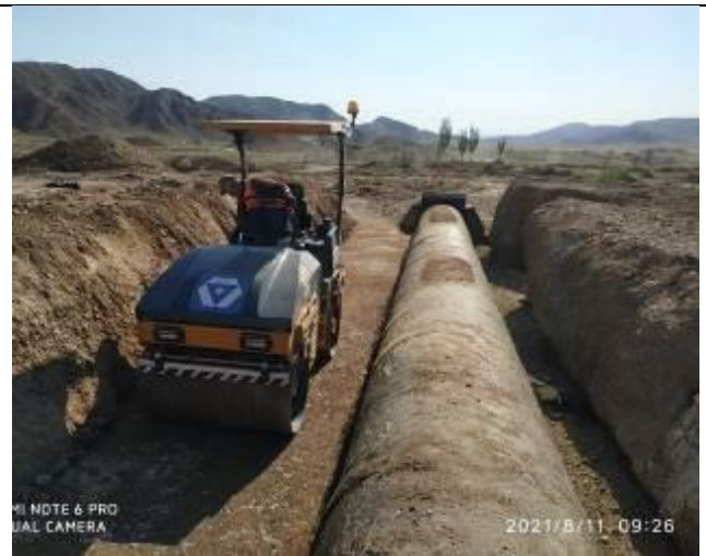
Photo 98. Lot 1. Compaction of soil backfill of culvert at km 20+670.
