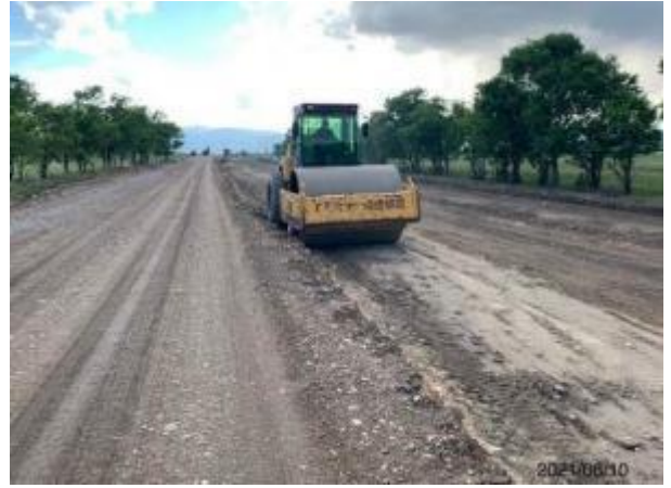
Lot 2. Section km 79+300. Photo 6 after tree cutting and road widening.
