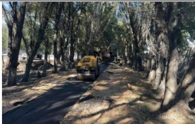
Photo 84. Sidewalk paving on km 2+050-2+414 LHS. September 2024.
