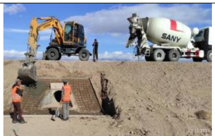
Photo 102. Lot 2. Slope reinforcement at culvert inlet km 71+800 LHS.
