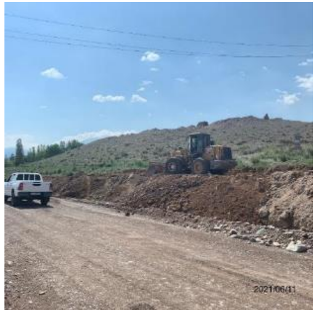
Photo 14. Lot 2. Removal of soil and vegetation layer from quarry site
