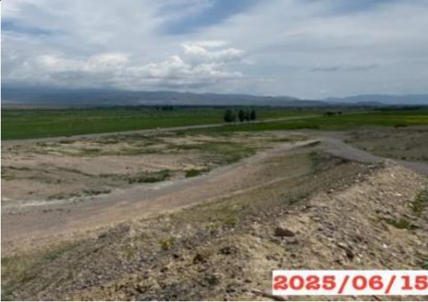
Photo 26. Dump of unsuitable soil at km 80+900, after reclamation
