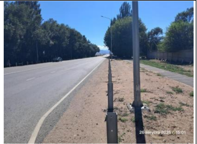
Photos 12, 13. Lot 1. Installation of additional guardrail for street lighting. August 2025.
