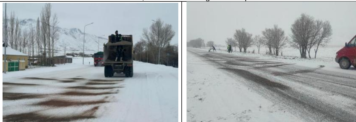
Photos 18, 19. Lot 2. Sprinkle of aggregate material
