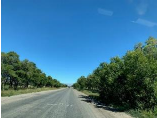
Lot 2. Section km 79+300. Photo 5 before tree cutting
