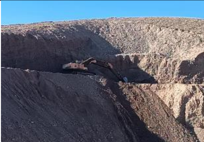
Photo 27. Quarry km. 75+400. Setting sides to a stable position.
