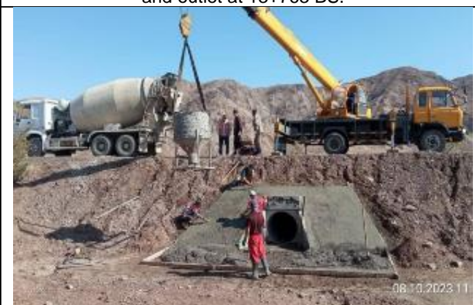
Photo 101. Lot 1. Concrete reinforcement of culvert inlet and outlet at 18+326BS.
