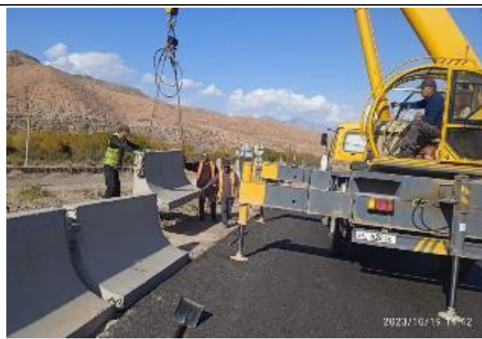
Photo 110. Installation of parapets at km.11+200.
