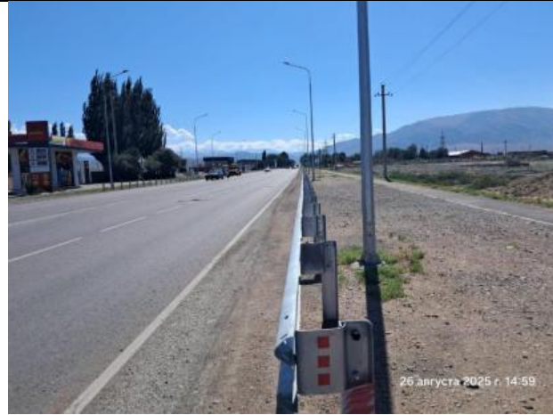
Photos 12, 13. Lot 1. Installation of additional guardrail for street lighting. August 2025.
