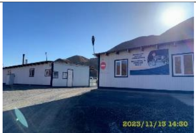
Photo 120. Lot 1. Accommodation Camp and Subcontractor's Office.
