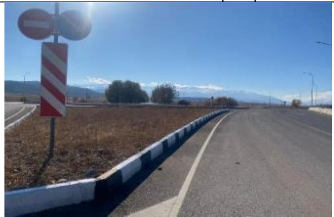
Photo 82. Lot 2. Roundabout at km 62+00.
