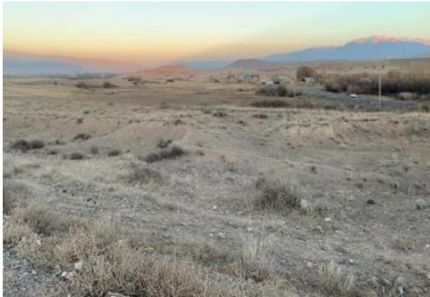
Photo 28. Lot 2. Site for the disposal of old asphalt at km 89+093 prior to its placement.
