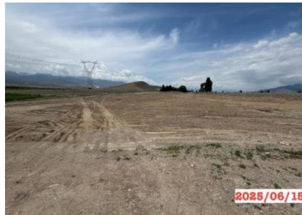
Photo 23. Old asphalt dump at km 70+180 LHS after reclamation
