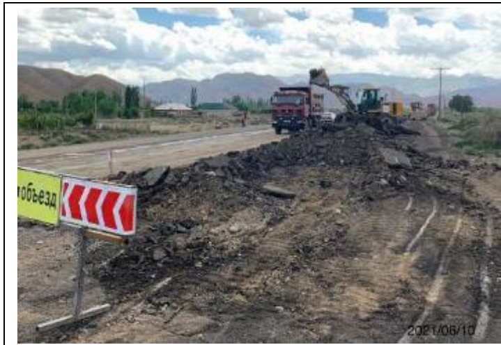
Photo 39. Lot 1. Scarifying and removal of old asphalt concrete at km.7+560 to the old quarry at km 7+100.
