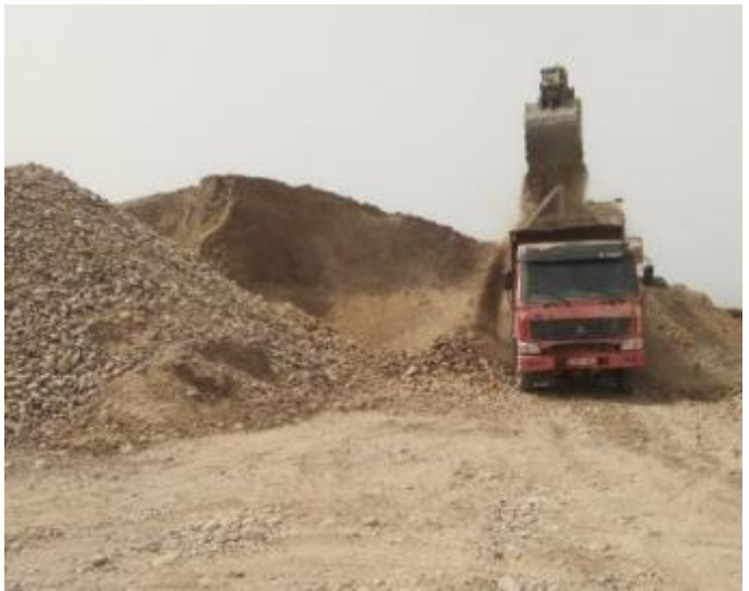
Photo 30. Loading of material at the quarry at km. 75+400.
