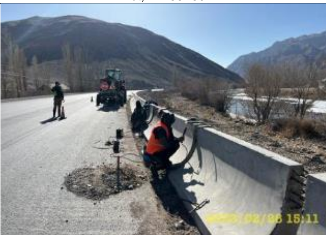
Photo 107. Lot 1. Assembly of installed parapets from km 14+000-15+000. February
