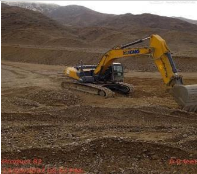
Photo 29. Quarry technical leveling at km 34+240 and bringing quarry slopes to a safe condition.
