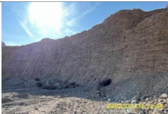
Photo 37. Quarry km 16+600. There is no stability of quarry sides: slope angle of quarry side is 90°, it should be 40-45°
