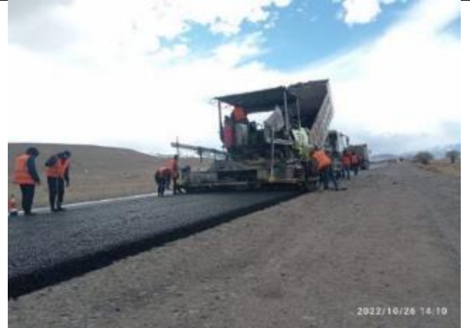
Photo 75. Lot 2. SMA arrangement km 81+675-82+000 RHS.
