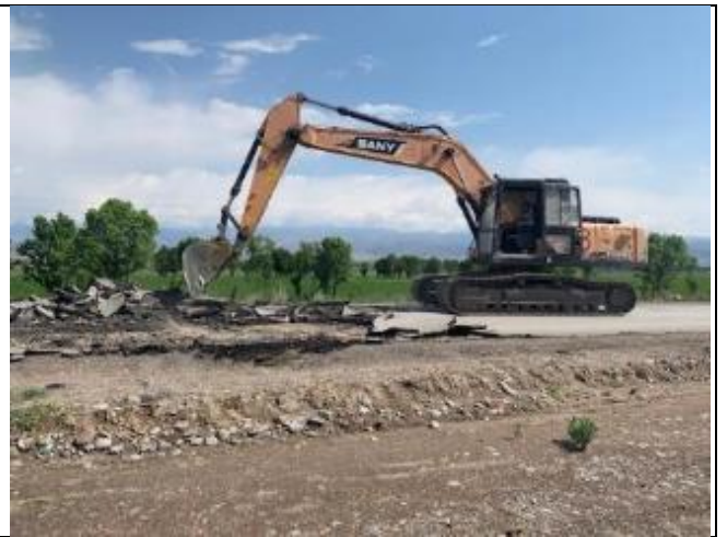
Photo 50. Scarifying of asphalt concrete pavement at km 74+550.
