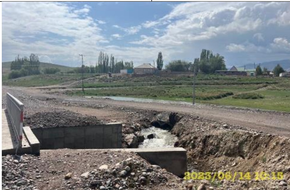
Photo 96. Lot 2. Bridge km 86+261. r. Sazdyn-Suus, bypass road.
