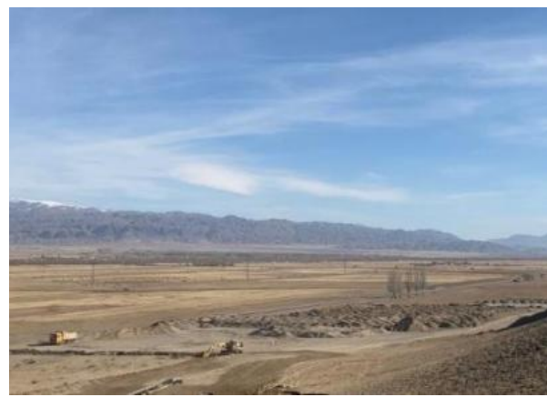
Photo 25. Dumping of unsuitable soil at km 80+900 during storage
