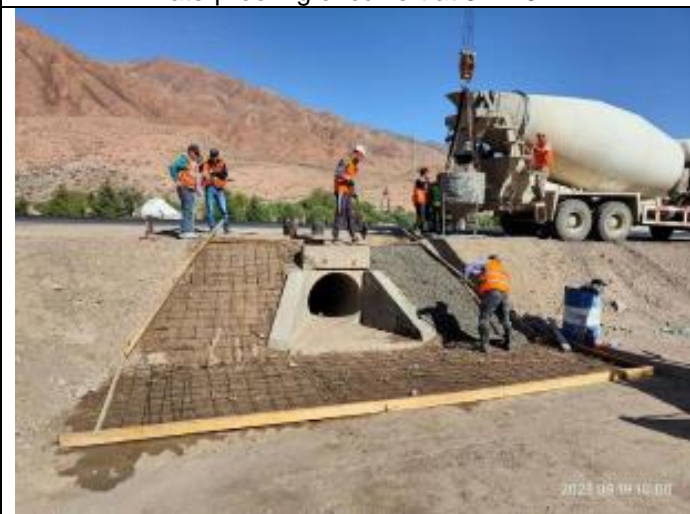
Photo 99. Lot 1. Concrete reinforcement of culvert inlet and outlet at 13+763 BS.
