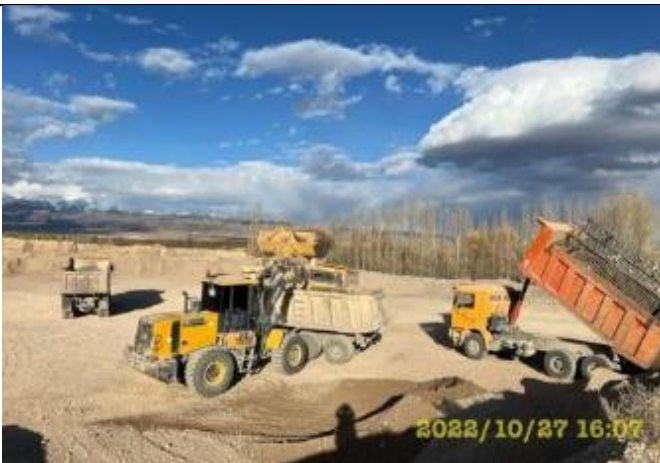
Photo 33. Quarry at km.75+400. The material is being mined, after it has been moistened.
