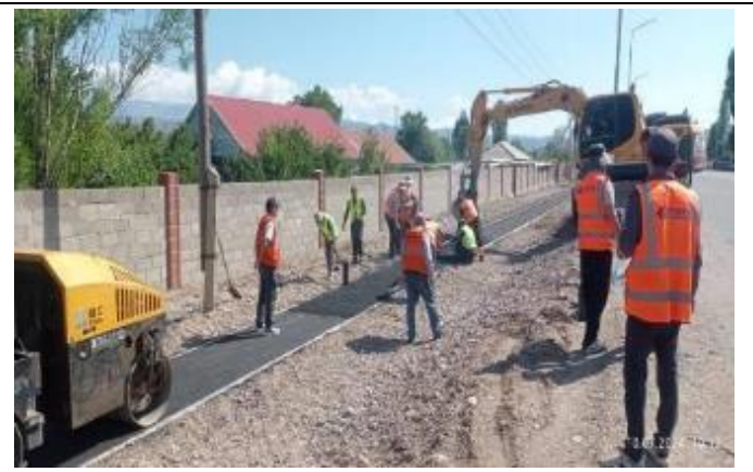
Photo 85. Lot 2. Sidewalk paving at km 70+100-70+740 LHS.
