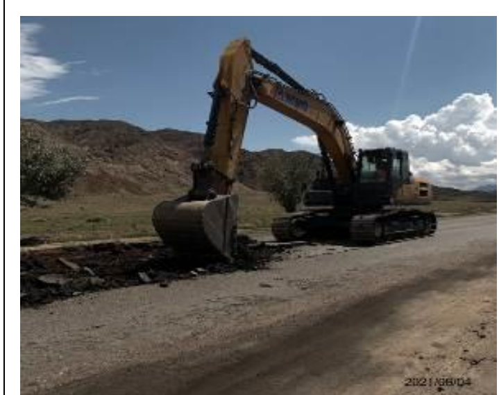
Photo 41. Scarifying of old asphalt at km. 17+500.
