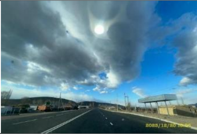
Photo 80. Lot 2. Road with new asphalt pavement.
