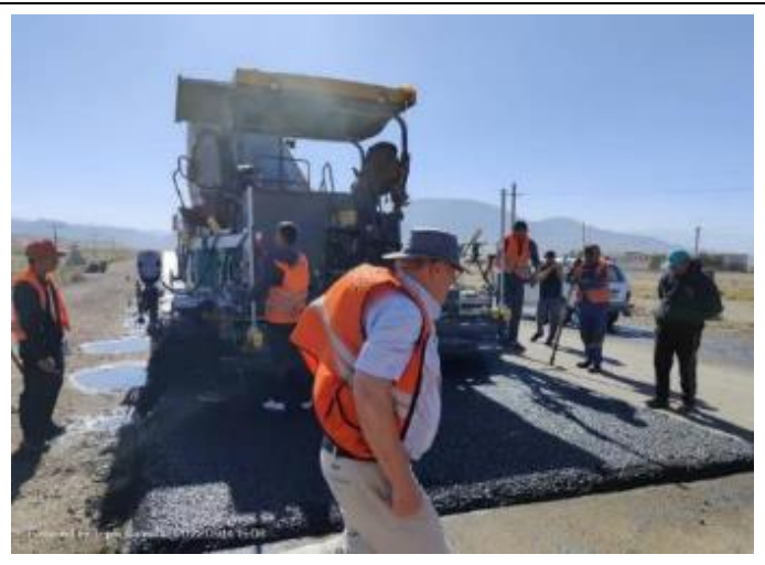
Photo 75. Lot 2. SMA arrangement km 81+675-82+000 RHS.
