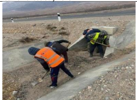
Photo 10. Cleaning culverts.
