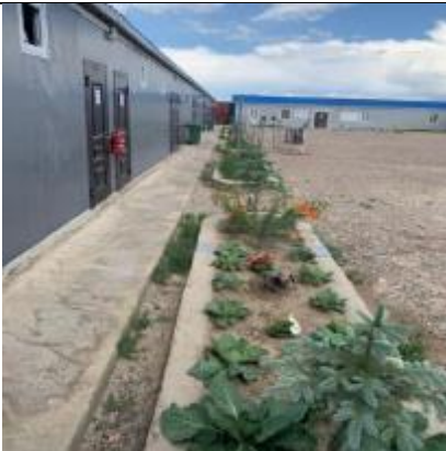
Photo 132. Contractor's camp. Accommodation rooms.
