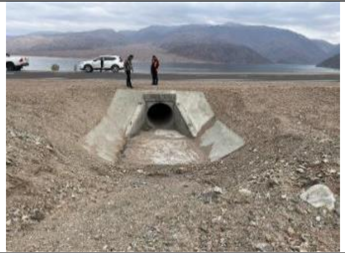
Photo 104. Lot 1: Culvert cleaning, km 33+869.
