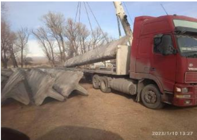
Photo 92. Lot 2. Removal of dismantled bridge slabs at km. 62+400.
