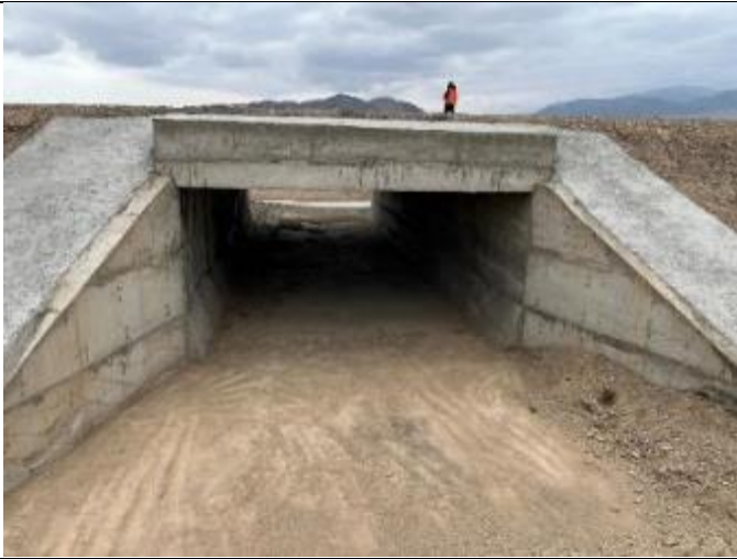
Photo 103. Lot 1, km 22+575, culvert cleaning.
