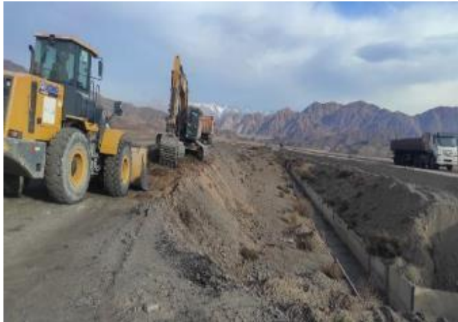
Photo 40. Lot 1. Scarifying and removal of asphalt from temporary bypass roads.
